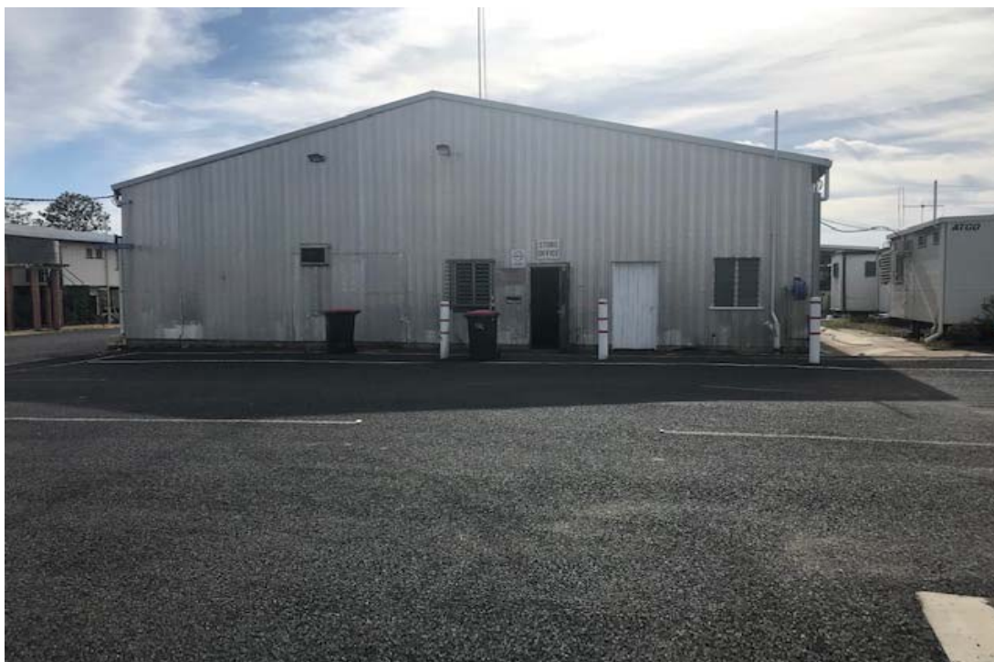
Photo 1 - Council Works Depot (Inglewood Stores Office)
