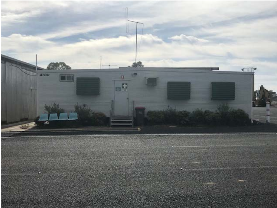
Photo 2 - Council Works Depot (Inglewood Supervisors Office/Lunchroom Donga)
