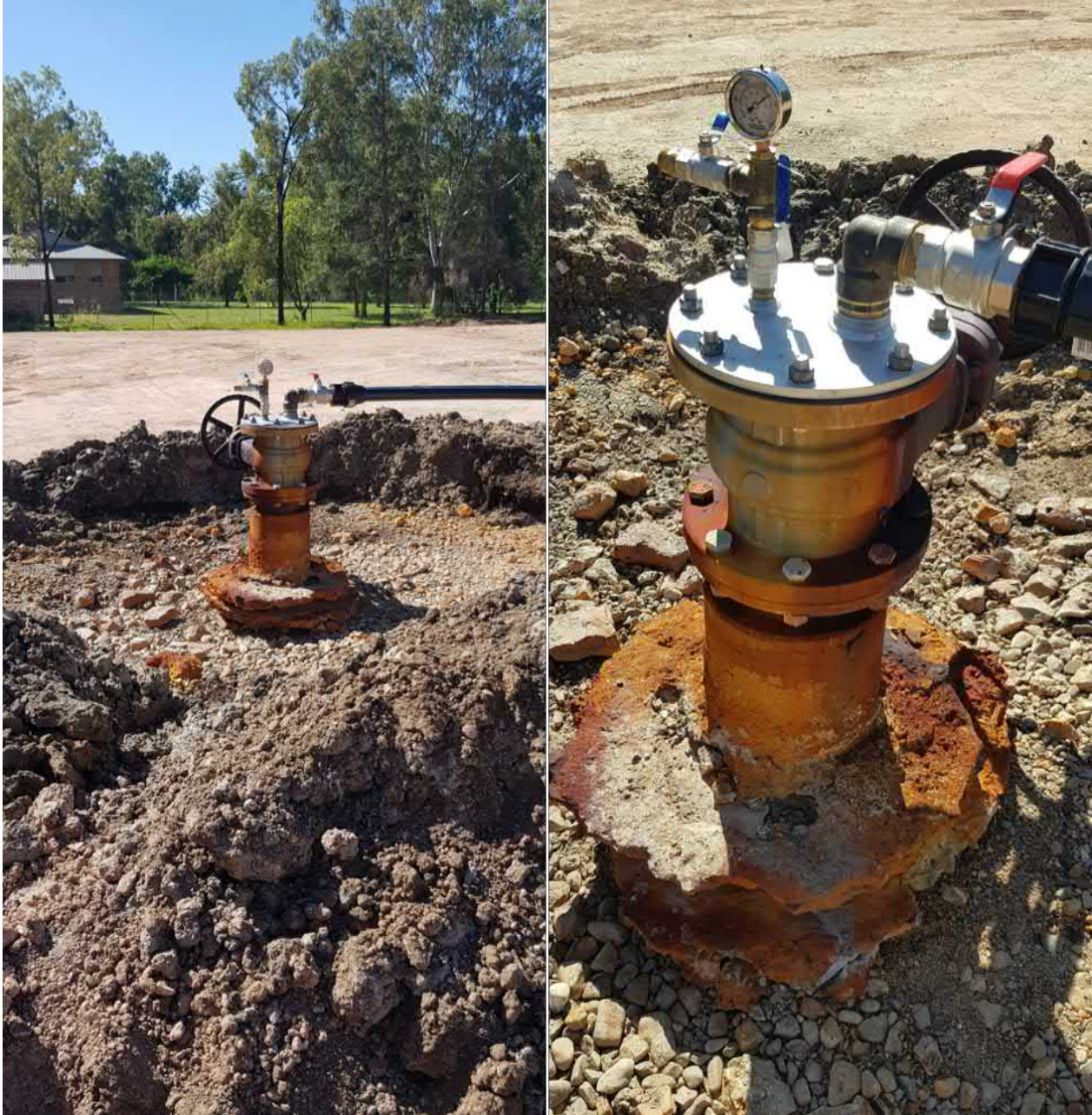
Figure 1 Images of Hutton bore installation (note iron staining suggests a high concentration of iron present, however the water quality data available suggests the concentrations are below aesthetic limits)
