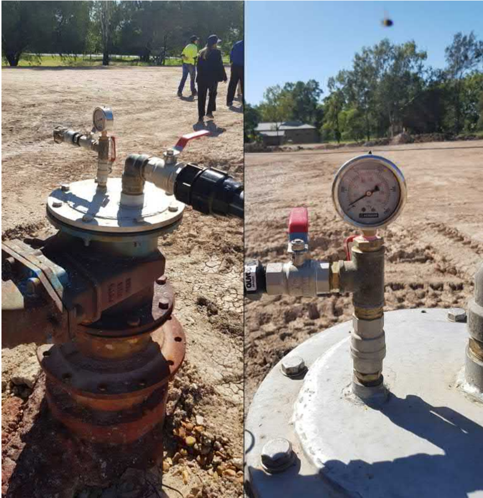
Figure 5 Images of Gubberamunda bore installation (note iron staining also noted on the bore shaft)
