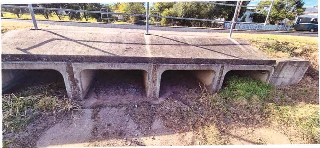
Figure 1-2 Culvert Crossing Under Cadell St Upstream of Site
